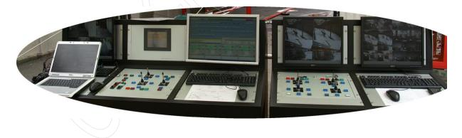
The system is designed for a multiuser environment. Through the redundant construction of the local network and a wireless LAN (WLA) it is possible to maintain the visualisations of the system in separate rooms.
